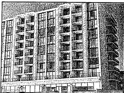
Figure 44 - Ocean-front condominium with continuous stand-off louvers extending full height of building. To prevent recirculation, dividers separate each floor level, and are also placed at each unit, near the upper edge of the condenser coil.
